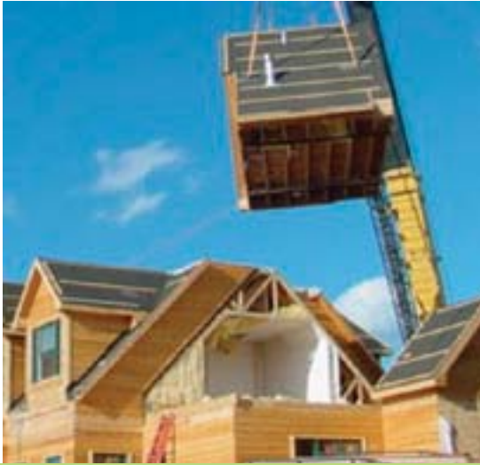
(Left) Five Oaks Homes in Colorado uses modular construction to build its prefab homes. Using this method, the homes are actually an assemblage of “boxes,” each containing its own wiring, plumbing and windows. (Middle and right) Sherie and Monte Pitt commissioned Deck House to assemble this prefab “custom” home for their hilltop Oregon property so it would highlight the surrounding mountain vista.
